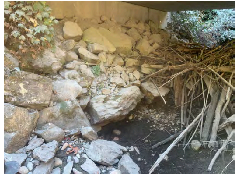
Right Bank Abutment when facing downstream
