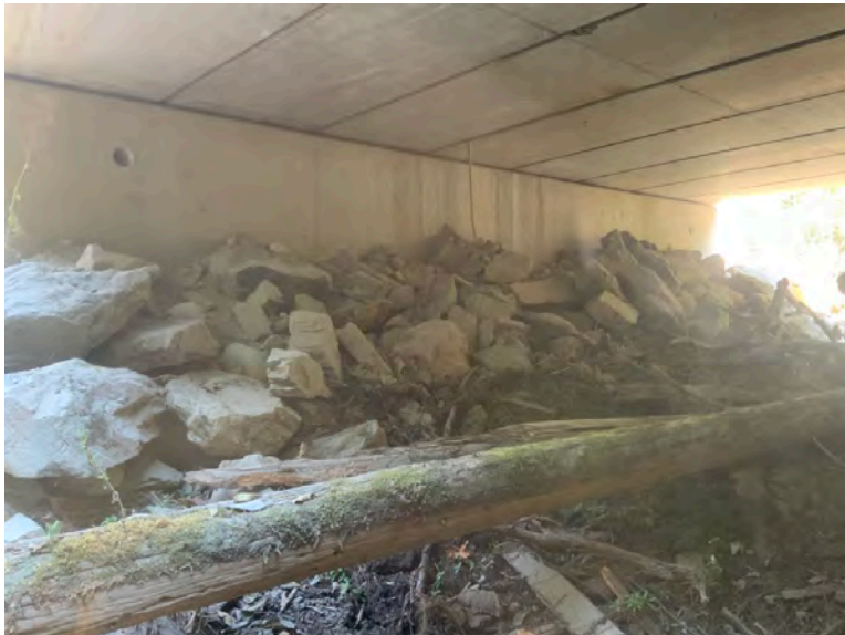
Left Bank Abutment when facing downstream
