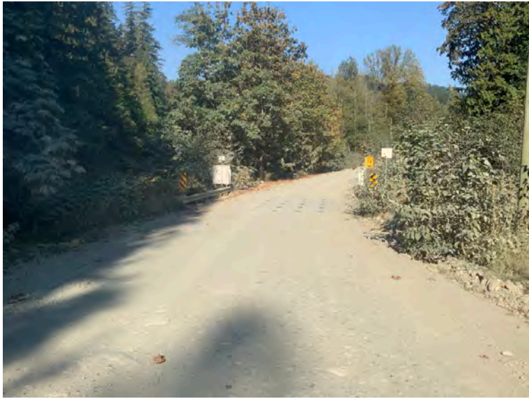
Approach from Left Bank when facing downstream
