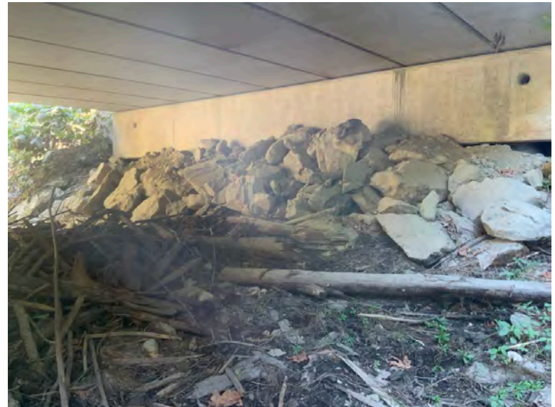
Right Bank Abutment when facing downstream
